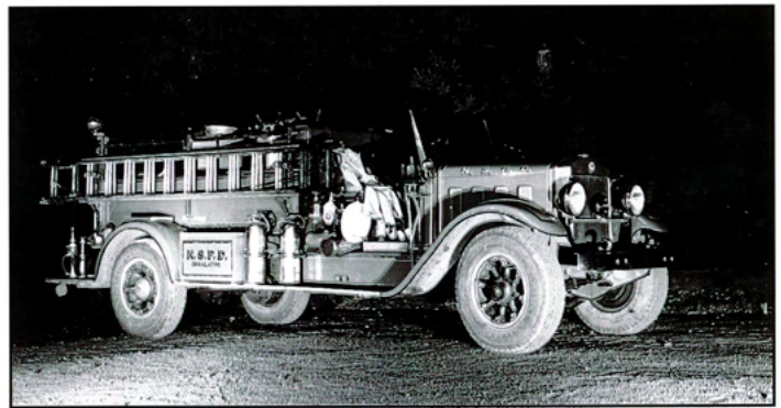
1933 Sanford "Buffalo" – Engine 1 was the department's first motorized pumper.
