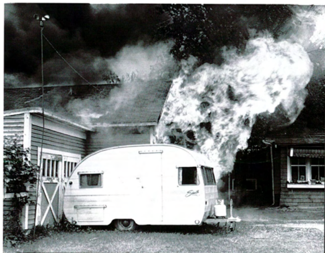
Garage fire at 306 South Main Street on June 20, 1961.
