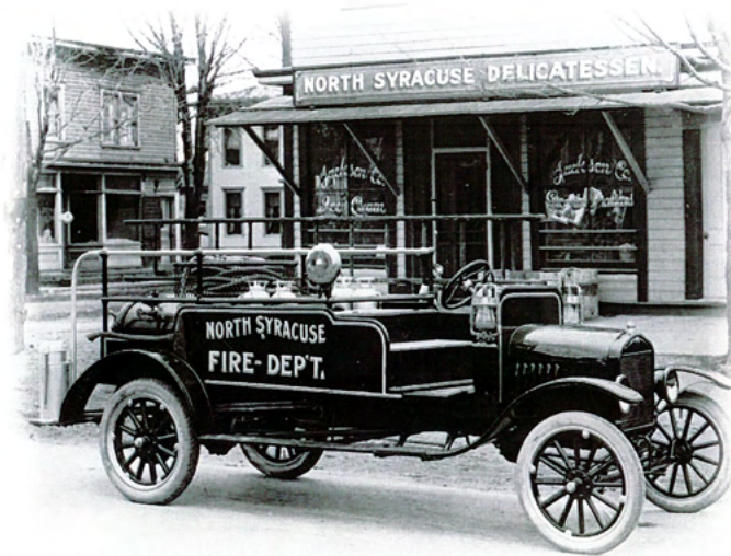
1921 Ford Model T Chemical Truck. The chemical truck held two 75 gallon tanks.
