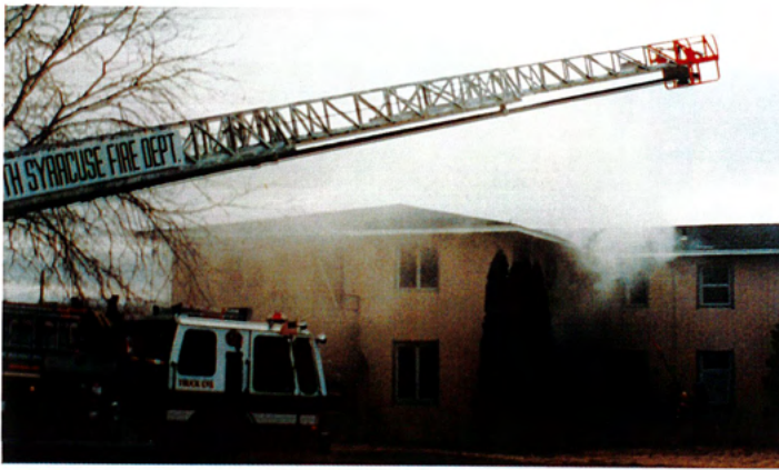
Fire at the Air Base Housing.
