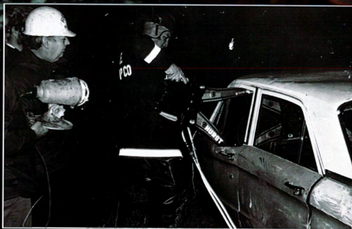
New Hurst tool training in the 1970's for vehicle extrication.
