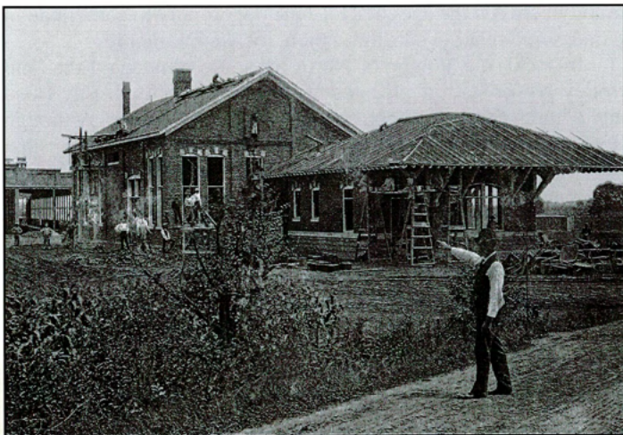
Above & below: South Bay and Church St. Trolley power station, which would eventually become North Syracuse Fire Station 1 in 1963.
