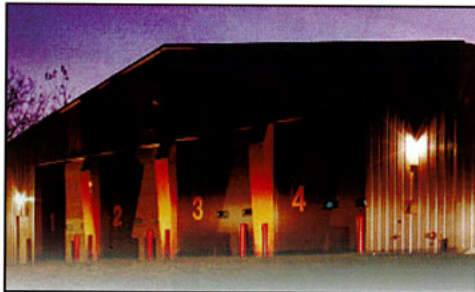
Current Station 2 at 70 General Irwin Blvd.
